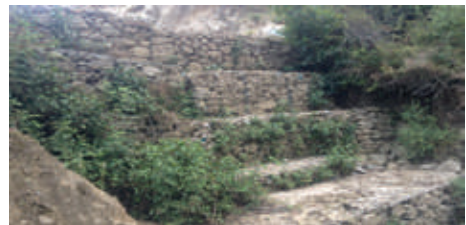
रिटेनिङ्गवाल (Retaining Wall)
